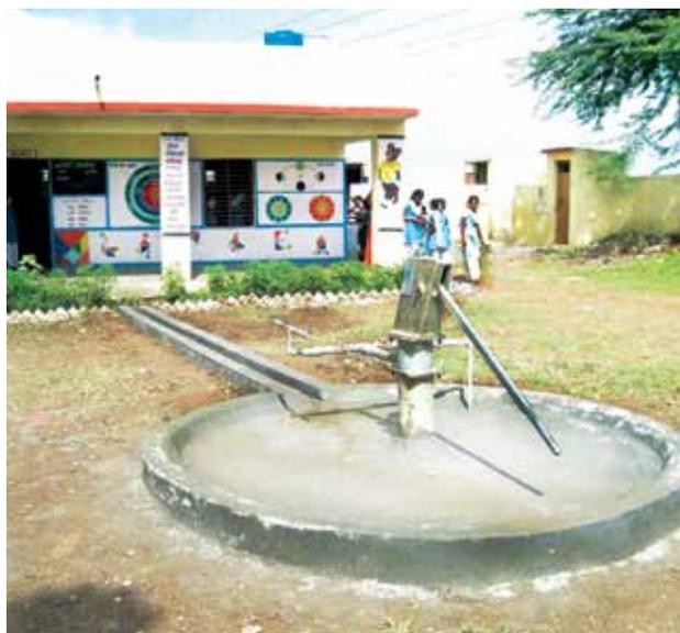
Findings of a validation study by UNICEF and RCEE established that upgrading of hand pumps to FLPs enhanced the availability of running water for toilets and handwashing in schools. The installation and maintenance of FLP was simple as it could be done at the local level. Contributions by the community and teachers in the installation and maintenance of the units showed a high level of acceptance to this technological innovation.
